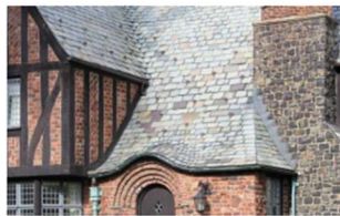
Slate hip roof with gabled projection and overhanging eaves of this Tudor Revival home at 140 Forest Avenue
