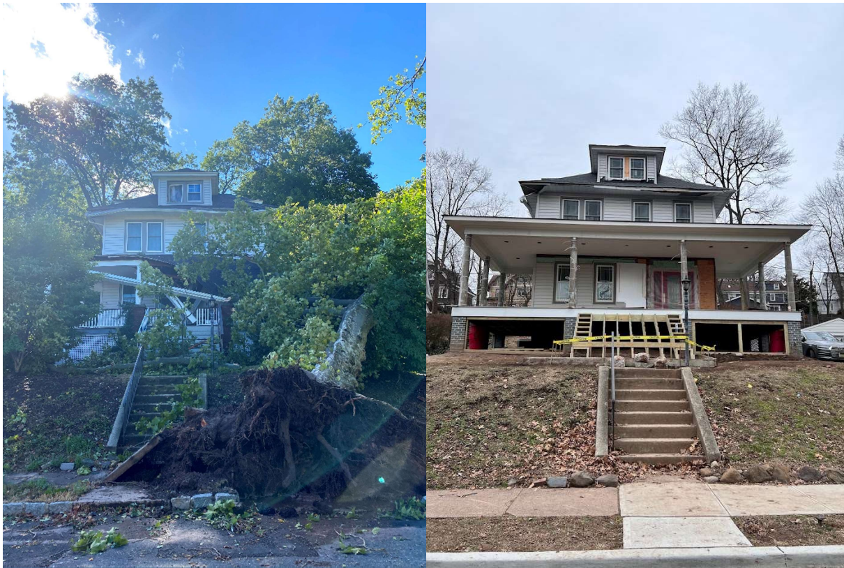
Photos of 2020 Hurricane Isaias storm damage at 38 Clinton Rd, and current progress
