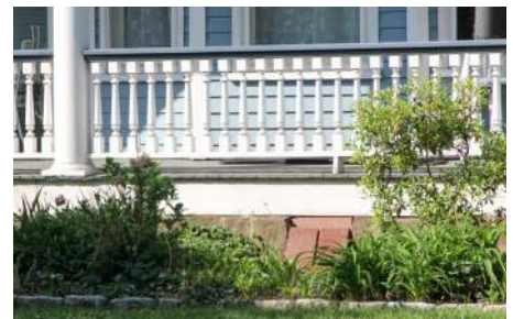
Some porches have stone foundations which support the wood frame and deck
