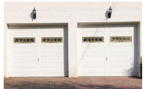
✗ Inappropriate contemporary garage doors
