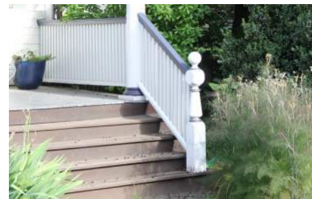
Stair railing terminates with a decorative newel post
