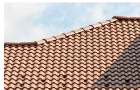
Limited instances of faux terra cotta tile are found on minimally visible and secondary roofs
