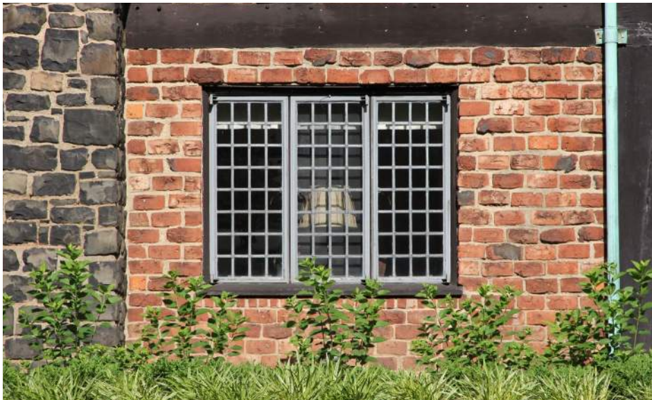
Multiple individual lites of glass set in a group of metal casement windows are a Tudor style feature of 140 Forest Avenue.
