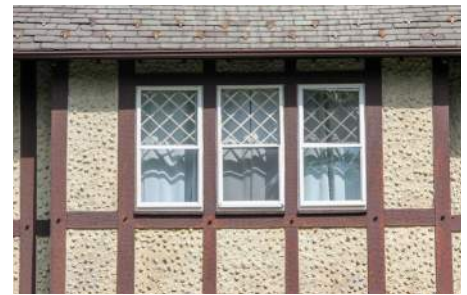
Pebble dash stucco between half-timbering
