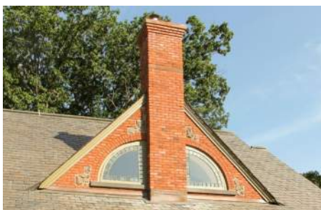
Gabled roof dormer with chimney at the Ridgewood Avenue Station
