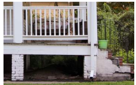
✗ Inappropriate open piers
