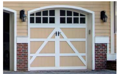
Garage doors reminiscent of a historic carriage house
