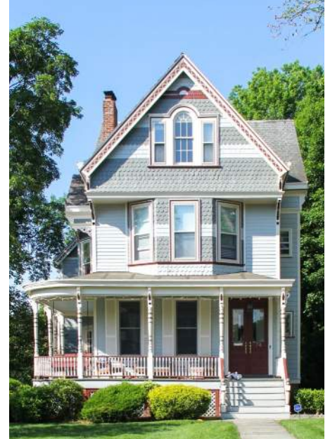
Queen Anne style homes feature a wide variety of wood siding and shingles.
