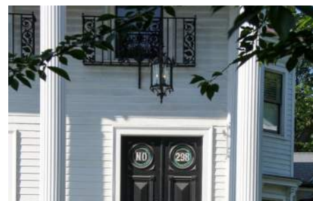
Light fixture suspended in double-height porch over front entry
