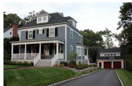
Even after expansion, the detached garage at 23 Douglas Road is subordinate to the primary building
