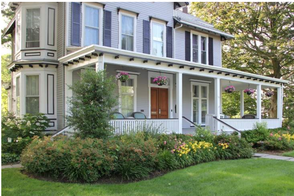
Bracketed box cornice and tightly-spaced balusters across the front porch are some of the Victorian details of 79 Forest Avenue
