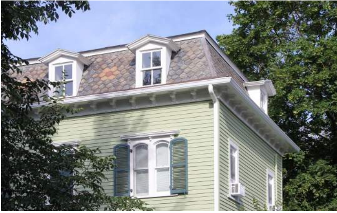
Second Empire style tiled mansard roof with gabled dormers at 50 Essex Avenue
