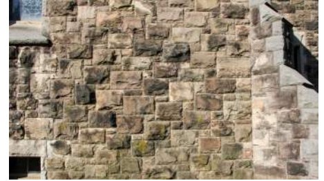
Glen Ridge Congregational Church ashlar
