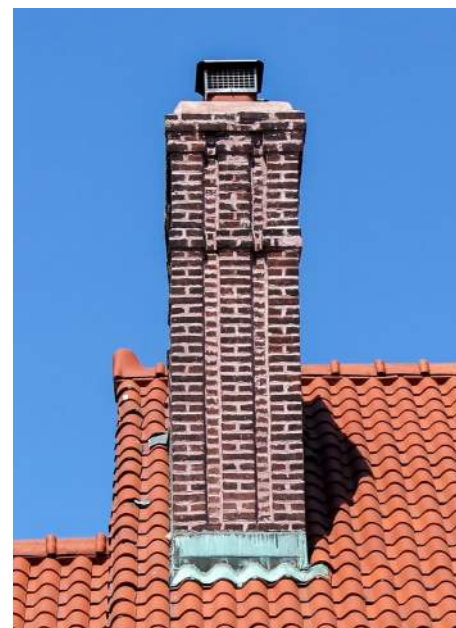
Patinated copper flashing at the base of a brick chimney
