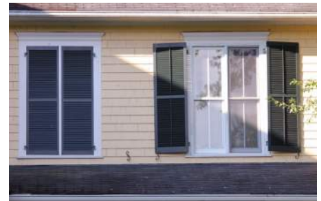
Operable shutters cover the window
