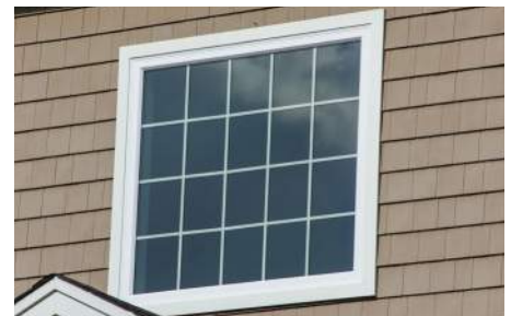
✗ Integral or snap-in muntin grilles with no profile on the exterior side are not appropriate
