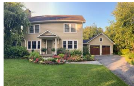
Attached garage is separated from the existing house with a hyphen, 70 Woodland Avenue
