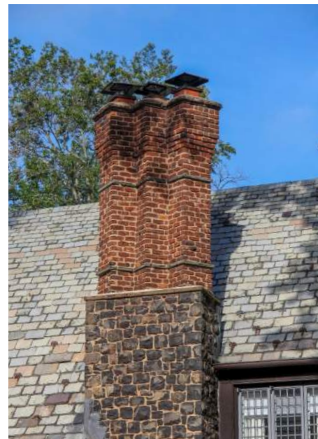
Brick and ashlar stone Tudor Revival chimney with multiple flues
