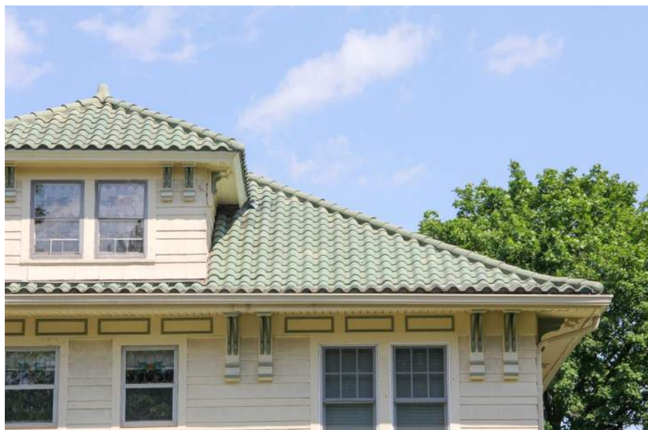
Scroll-sawn projecting brackets support the eave
