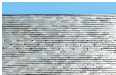
Slate varies in color, shape, texture, and details. Selective in-kind replacement from the same geologic formation is appropriate.
