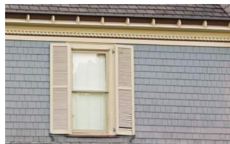
The small open gaps between wood shingles, called keyways, are essential to a well-performing enclosure.
