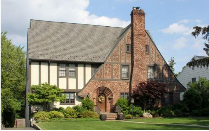
Tudor Revival homes typically combine brick and stucco with half-timbering
