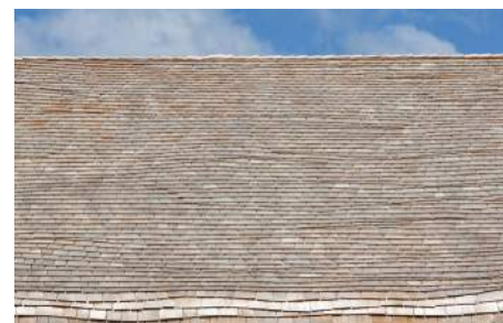
Wood shingle can be replaced with dressed wood shingle. The use of pressure-treated fire-resistant wood shingles is appropriate.
