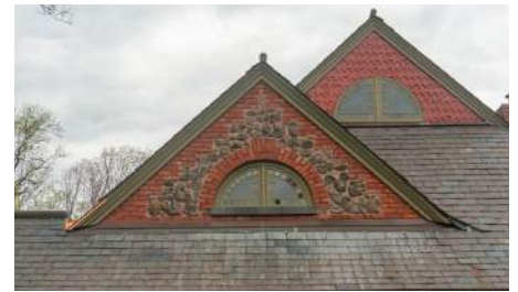
Ridgewood Avenue Station decorative masonry gable end
