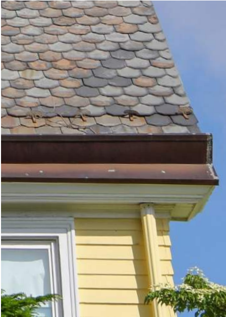
Lined pole gutter
