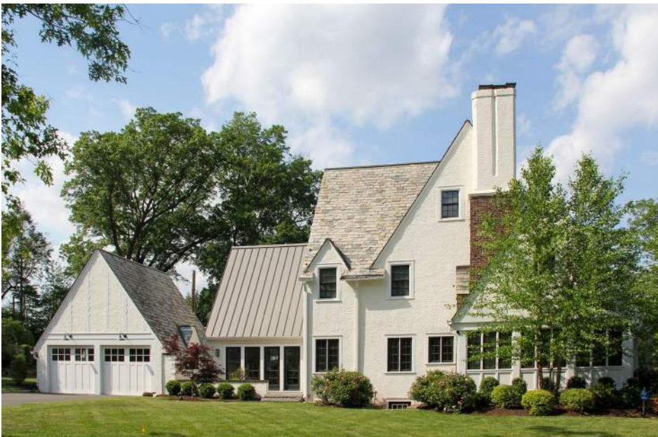
The side addition is differentiated from the original house through a change in roof material, 518 Ridgewood Avenue
