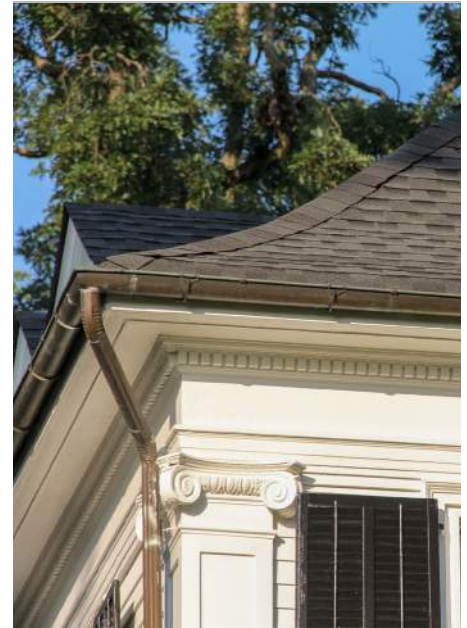
U-style copper gutter
