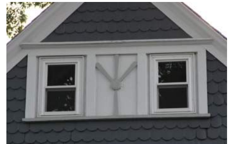
✗ Removing a window opening on a primary facade is not appropriate
