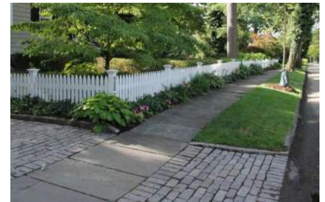
Bluestone sidewalk continues through cobblestone driveway skirt
