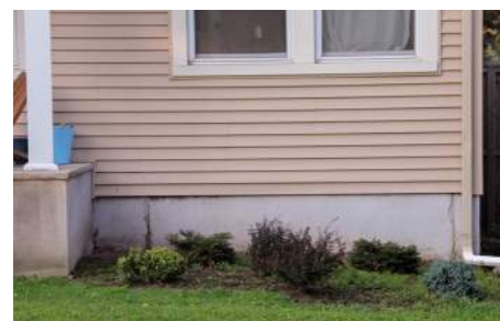
✗ Inappropriate exposed concrete foundation
