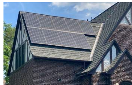
✗ Visible solar panels over a character-defining roof form diminish the historic building's integrity
