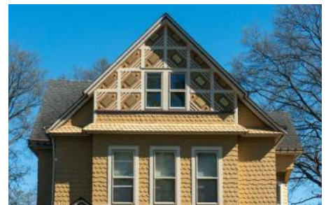
Wood shingle patterns and incised ornament on the gable end
