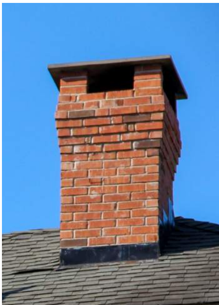
Chimney cap with corbeled brick
