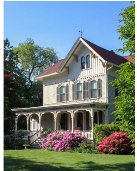
Patterned wood siding and decorative trim at 316 Washington Street
