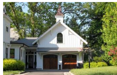
The varied massing of 298 Washington Street was able to accommodate an attached garage with cupola
