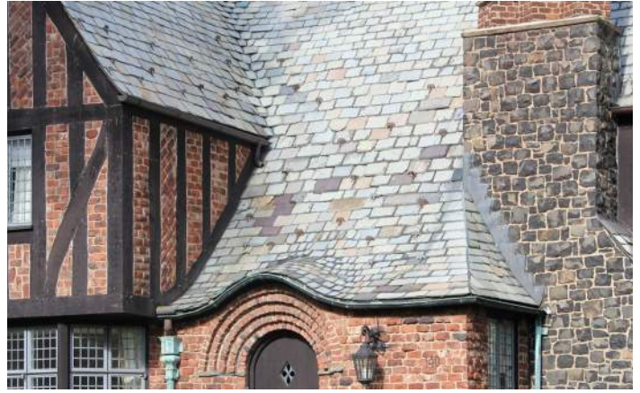
Slate hip roof with gabled projection and overhanging eaves of this Tudor Revival home at 140 Forest Avenue
