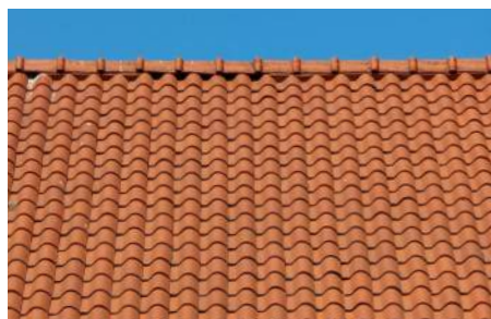
Terra cotta tile and clay should be preserved whenever possible. Selective in-kind replacement is appropriate.
