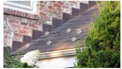
Metal snowguards and flashing
