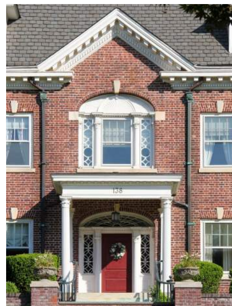
Symmetrical trabeated front portico of a Colonial Revival style house
