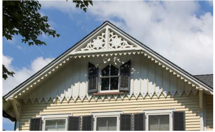
Decorative wood bargeboard and trim
