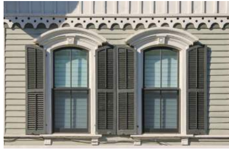
Pair of arched windows with round pediments and louvered shutters
