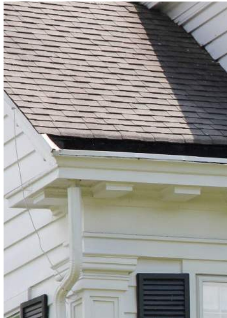
Built-in lined gutter
