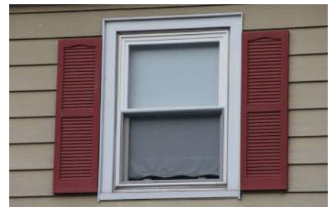
✗ Reducing the historic daylight opening of a window is not appropriate
