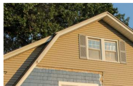
X Vinyl siding is not an appropriate siding treatment and should be removed
