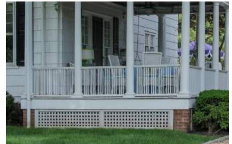
Framed square lattice below tightly-spaced balusters
