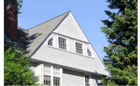
Wood shingle siding
