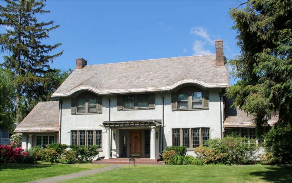
Thatch-like roof comprised of steam-bent cedar wood shingles at 388 Ridgewood Avenue
