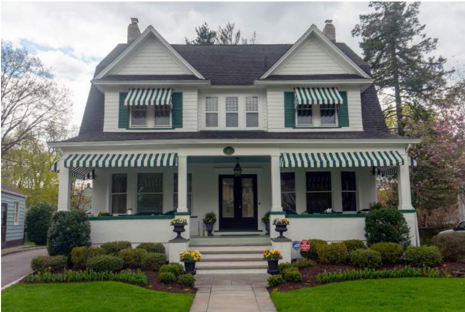
Awnings were added to 14 Rudd Court after an inappropriate glass enclosure was removed from the front porch
