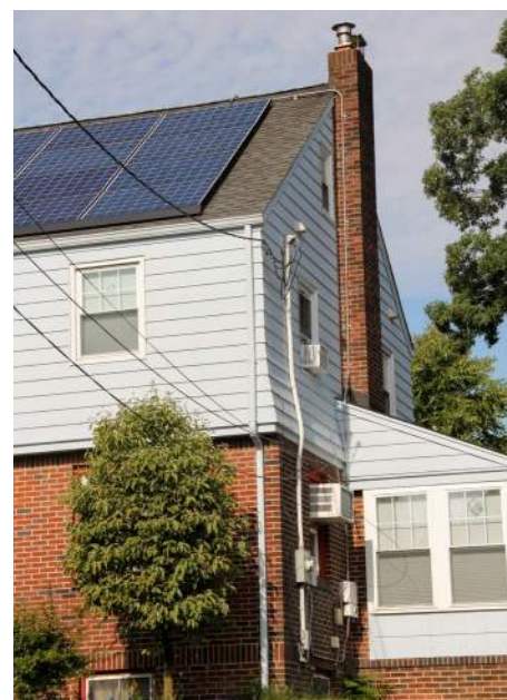
✗ Incidental utility equipment should not be visible
