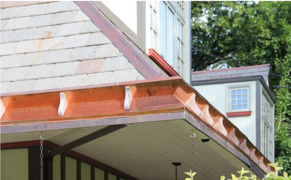
Copper flashing-lined pole gutter system at the former Benson Street Station.
