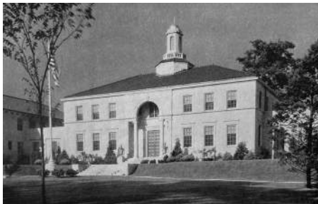
The Glen Ridge Municipal Complex was built in several phases between 1918 and 1931
