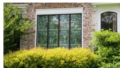
Protective glazing on the exterior side of stained glass at 298 Washington Street
