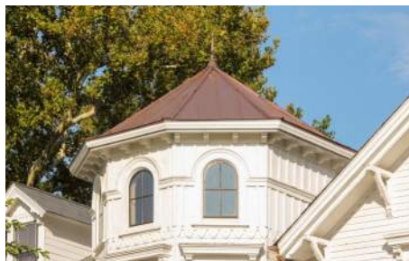
Metal roofs should be replaced to match the type, appearance, trim, and articulation of the original. Copper and painted terne are typically appropriate materials.
