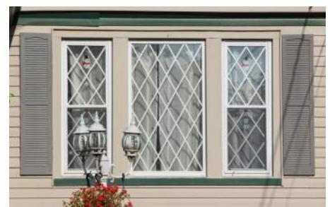
✗ Inappropriate narrow shutters fixed to the wall
