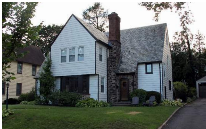
124 Stonehouse Road with stucco and half-timbering concealed by metal siding, prior to restoration project
