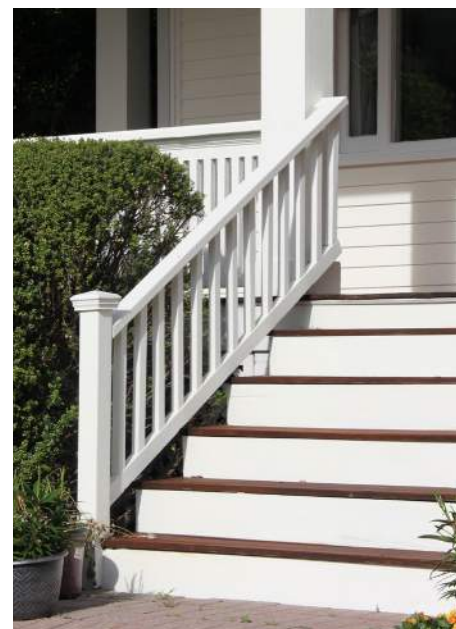
Railing with tightly-spaced balusters and newel post
