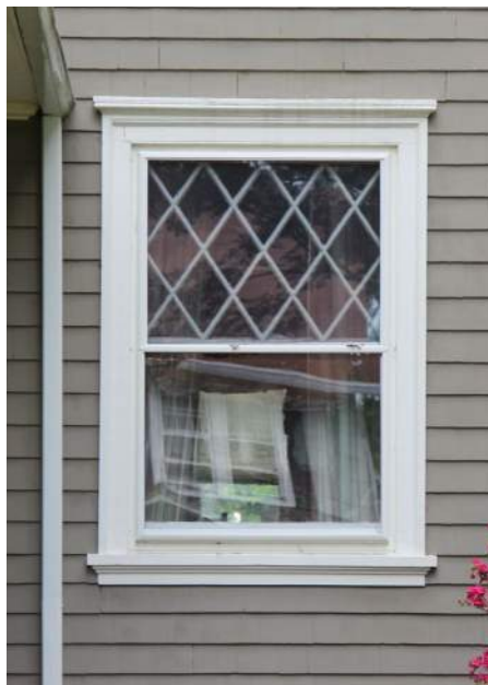
Properly-sized storm windows allow visibility of the upper sash diamond lattice
