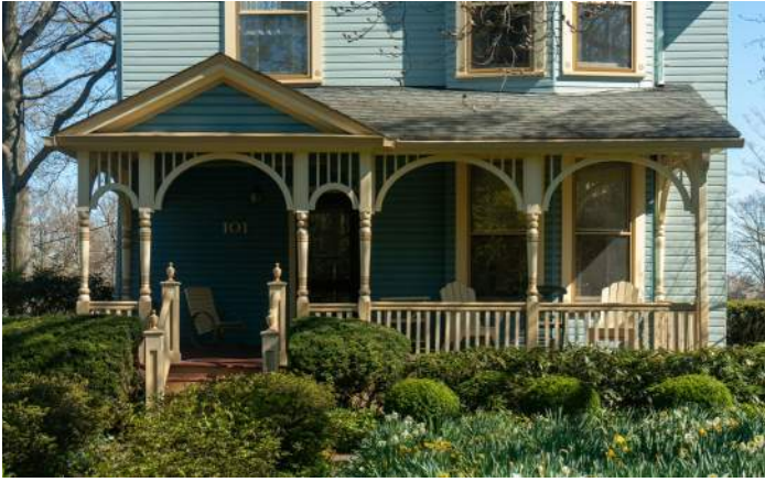
Wood spindlework porch
