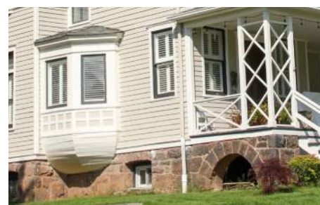
Foundation is articulated under front porch
