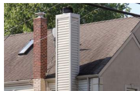
✗ Inappropriate chimney covered with vinyl siding
