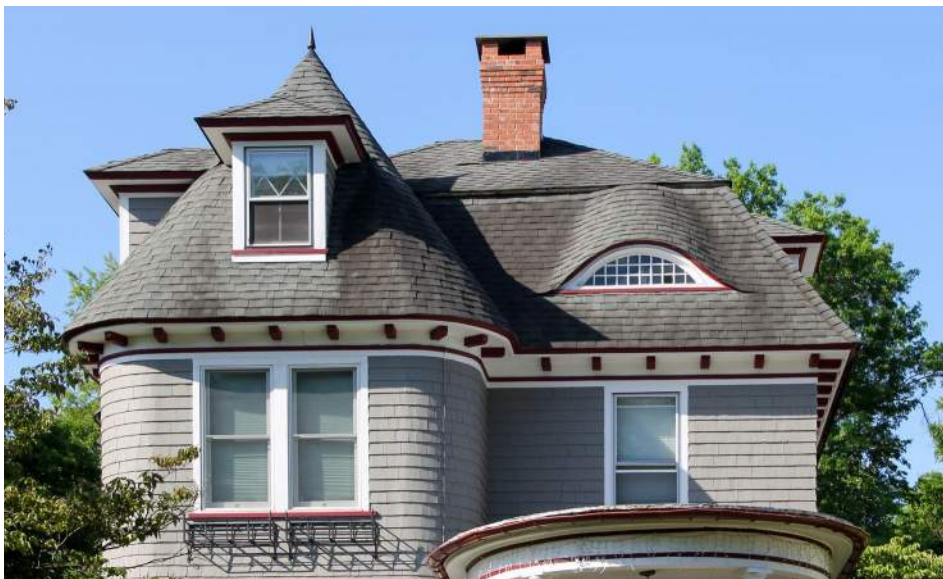
The complex hip roof with eyebrow dormer is an important character-defining element of this Queen Anne style house at 20 Winsor Place.
