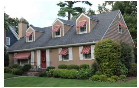
Awnings installed in a reversible manner
