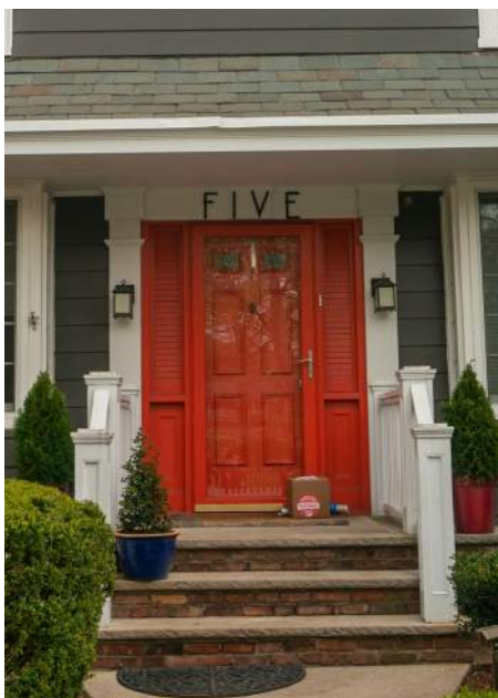
Low profile storm door finished to match
