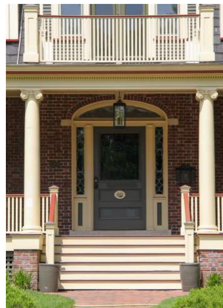
Simple light fixture between ionic columns
