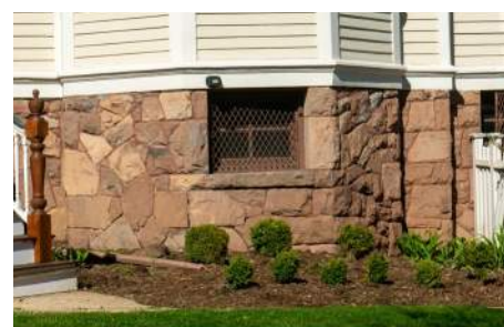
Rubble stone foundations are common in early Glen Ridge homes
